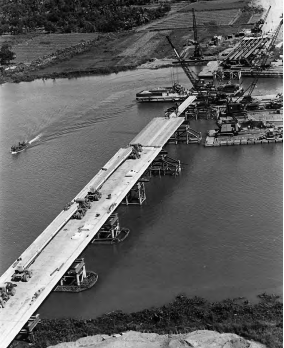
The Phu Cuong Bridge under construction
